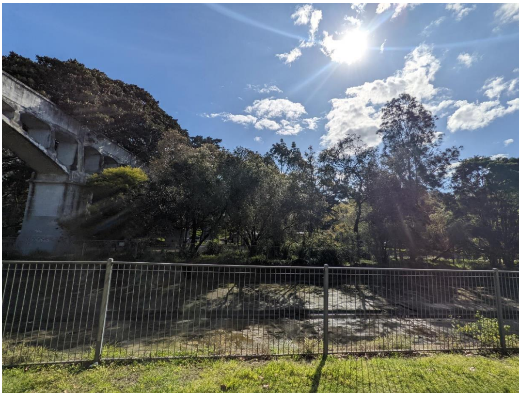
Figure 12: The view from the rear of the subject site, facing west
