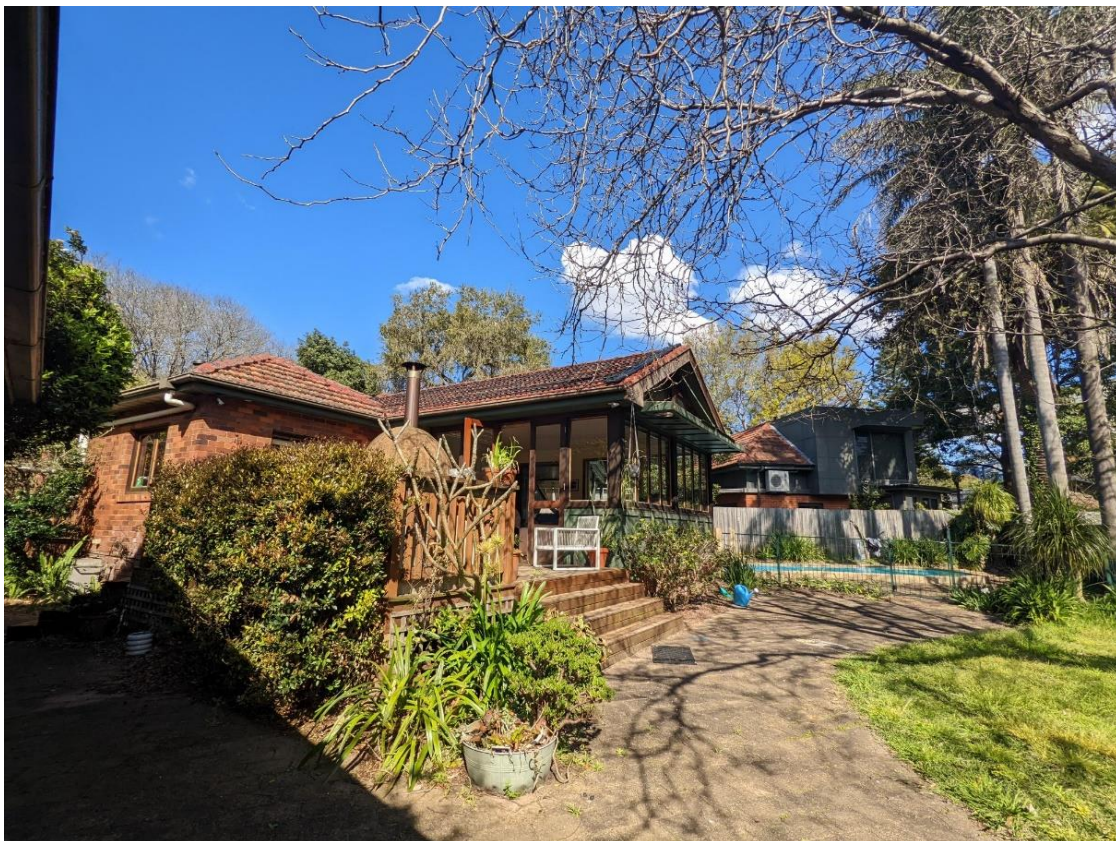
Figure 4: The rear of the subject site viewed facing south east
