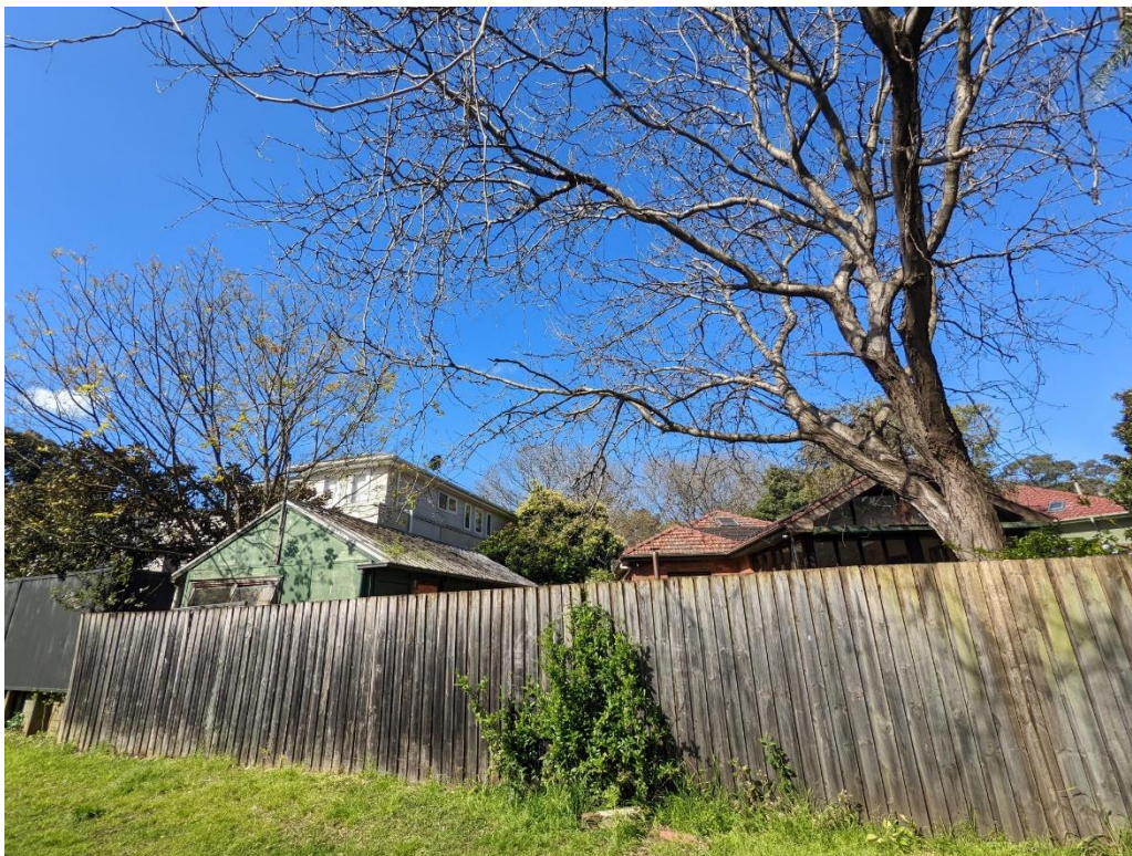
Figure 10: The rear of the subject site viewed from the public reserve facing north east
